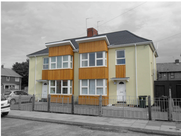
Figures: (1) Bay Window Pod by Datum being installed at the YHN Greenford Road 'Retrofit for the Future' site in Newcastle with (2) completed semi detached properties. (3) Roof Pod by Envirohomes Ltd being installed at the East Midlands Housing Association terraced property at (4) Cottesmore Road, Leicester.
